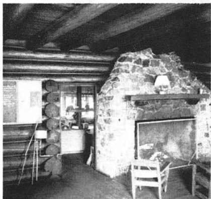
Exterior and interior views of Snoqualmie Lodge. (photos by Millspaugh)
