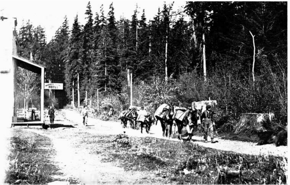
Upper—Suspension bridge over Diablo Canyon, Skagit River Lower—Pack Train leaving Marblemount for Upper Skagit Mt. Baker National Forest Photographs—circa 1913
